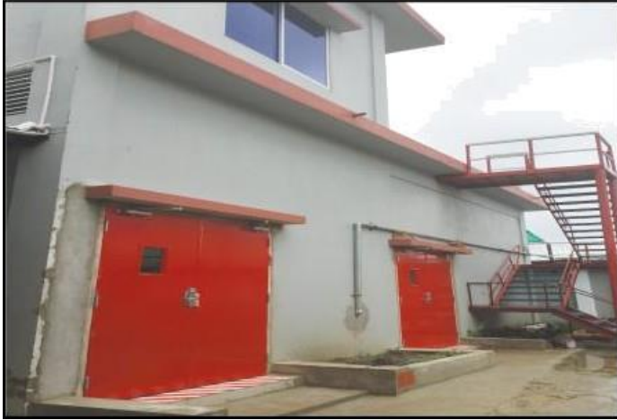
Compressor room (55 kg.)
